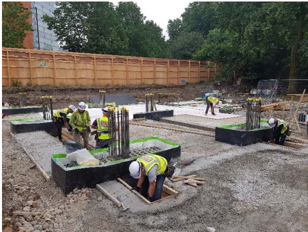
Construction of foundations to the future reading room
